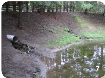
Photos 6 and 7. Ponds with large bare spots or low vegetation density on pond bottom or side slopes.
