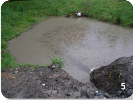
Photo 5. Pond with excessive sediment deposition.
