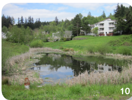
Photo 10. This permanent pool of standing water is a sign of minimal soil and water contact time.
