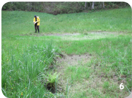
Photos 6 and 7. Ponds with large bare spots or low vegetation density on pond bottom or side slopes.
