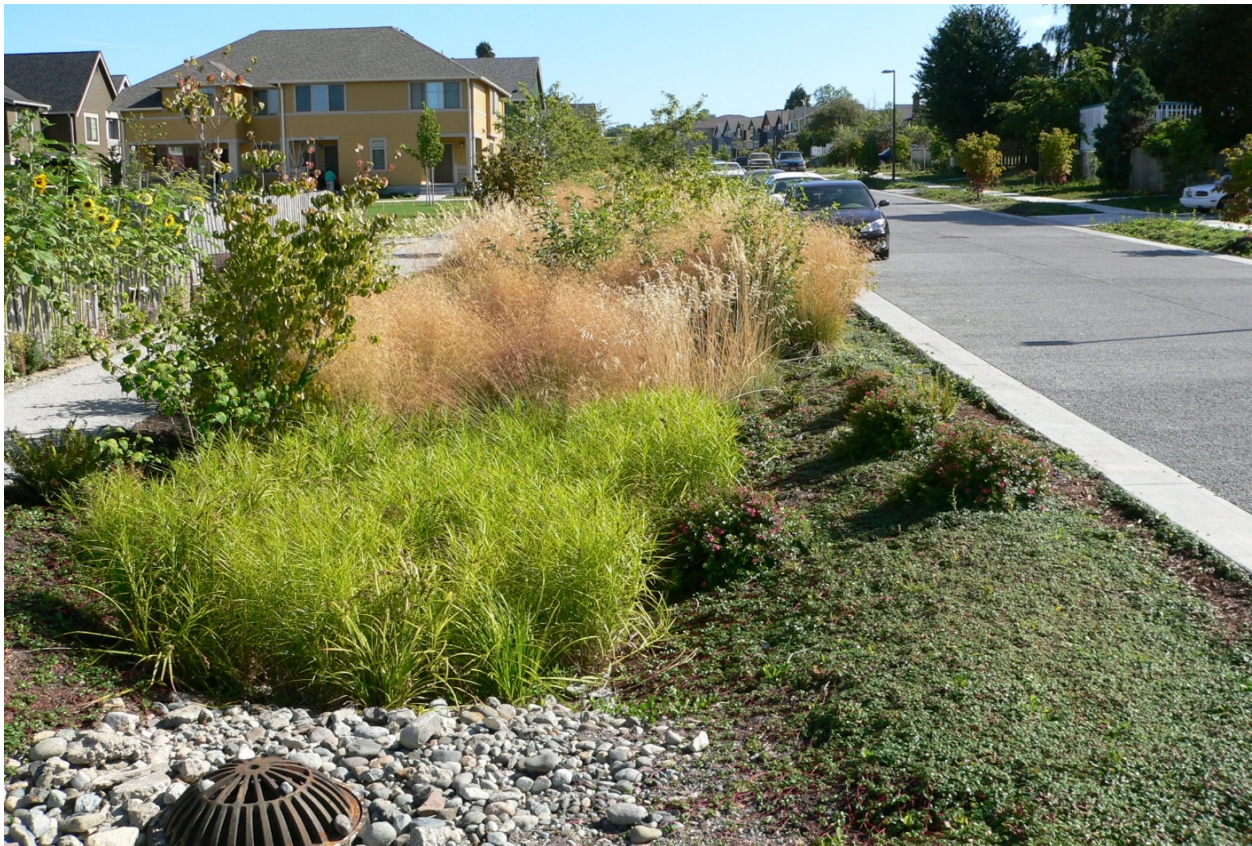
Figure 1. Typical Bioretention Application.
