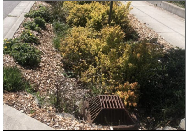
Figure A-16. Typical T117 Bioretention Cell.
