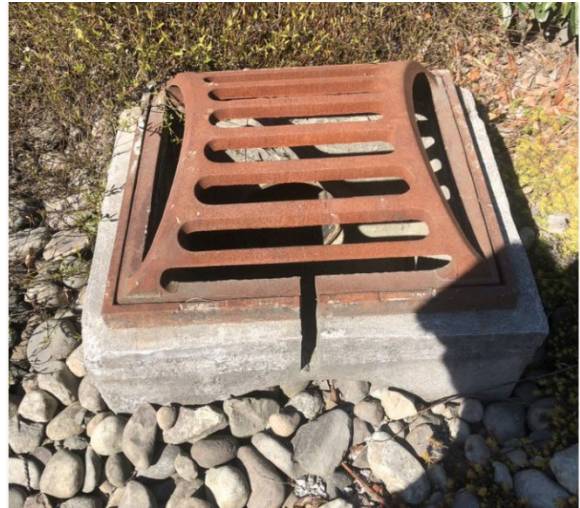
Figure A-10. Typical Overflow Structure and Notch.
