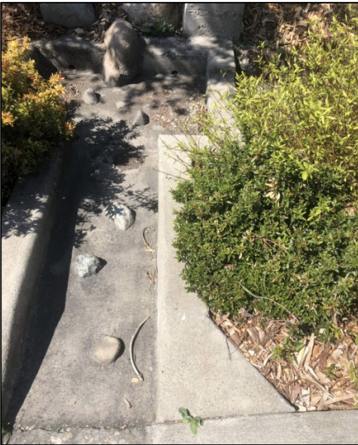
Figure A-17. Typical T117 Presettling Cell.
