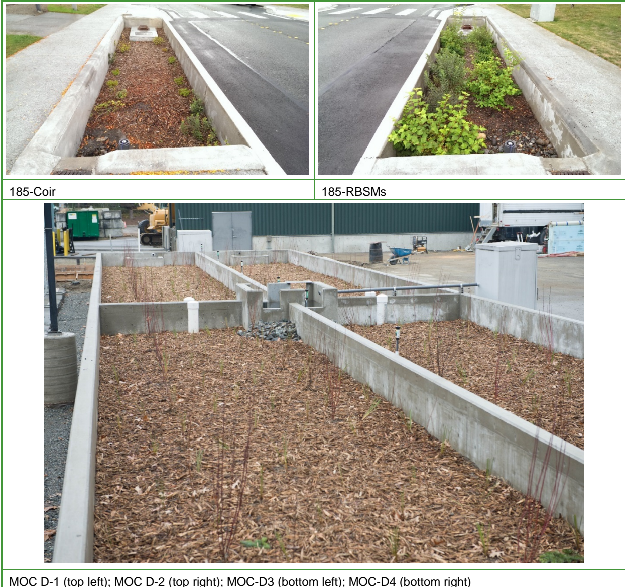
Figure 4. Photographs of the MOC and 185th Bioretention Swales.
