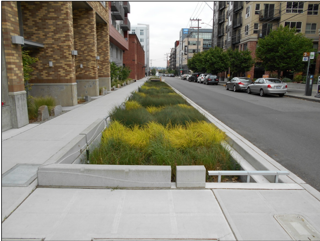
Figure 3. Photograph of Swale 2 (looking north).
